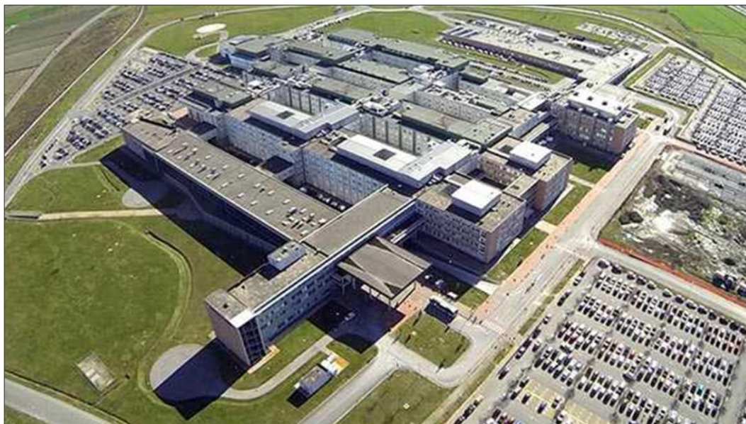
Figure 2. View of the Sant'Anna hospital of Cona (Italy).
